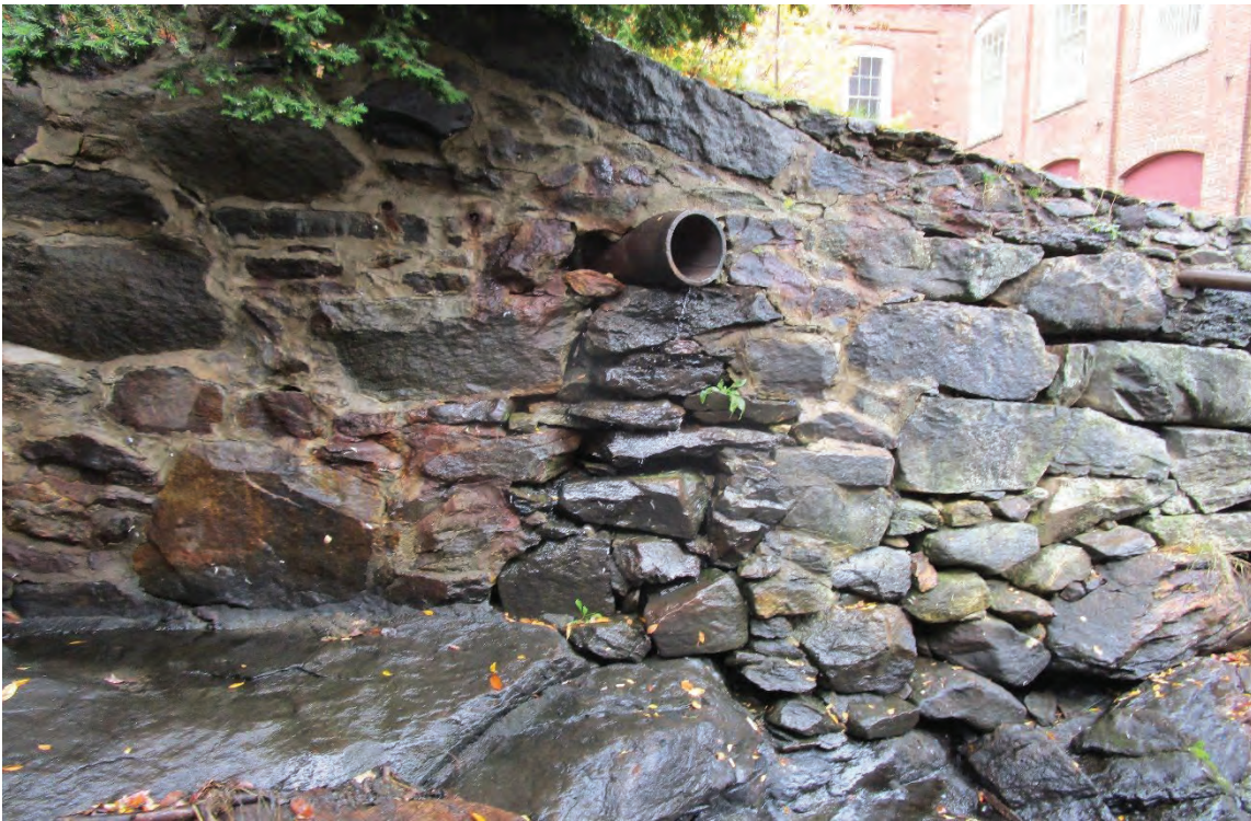
Photo 22: View northwest of the existing masonry wall. 10/16/2022.
