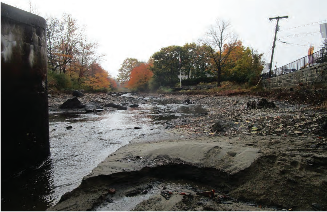
Photo 16: View south/upstream of the Contoocook River during drawdown conditions. 10/16/2022.
