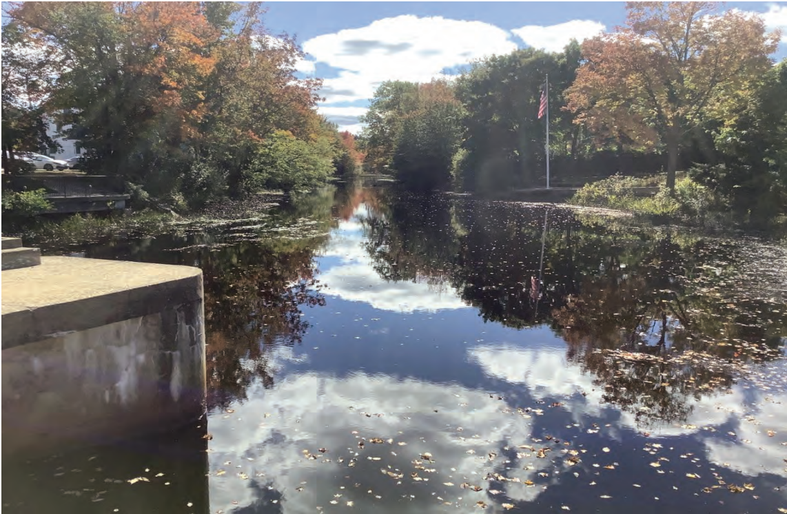
Photo 7: Upstream view south of the Contoocook River, taken from the US 202/Main Street Bridge. 10/07/2021.
