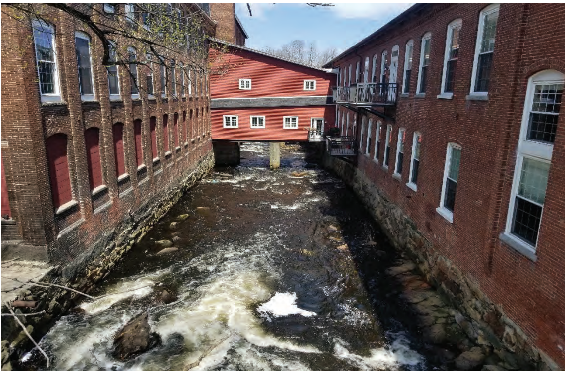
Photo 20: View northeast of the channelized portion of the Contoocook River downstream of the Site between the old mill buildings during normal flow conditions. 05/05/2022.
