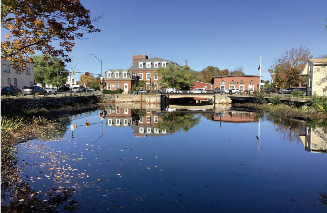
Photo 9: Downstream view north of the US 202/Main Street Bridge over the Contoocook River. Note the constructed walls on either side. 10/07/2021.
