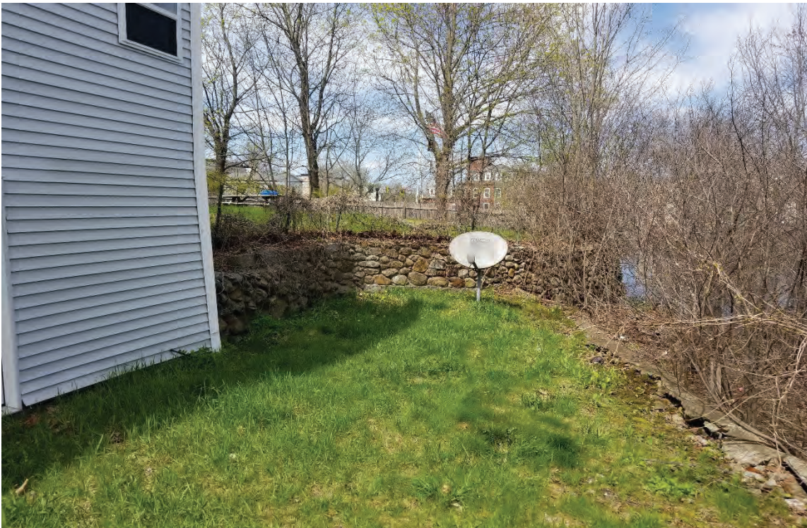
Photo 24: View north of the retaining wall on NHDOT Parcel #11. 05/05/2022.
