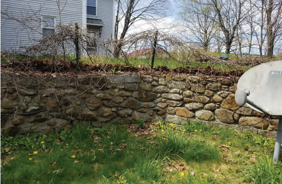
Photo 25: Closeup view northwest of the retaining wall on NHDOT Parcel #11. 05/05/2022.
