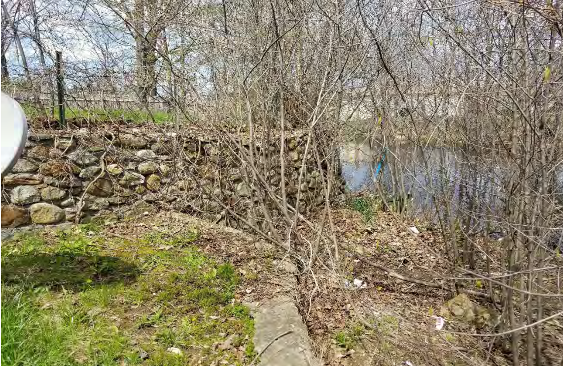
Photo 27: Close-up view north of the retaining wall on NHDOT Parcel #11. 05/05/2022.
