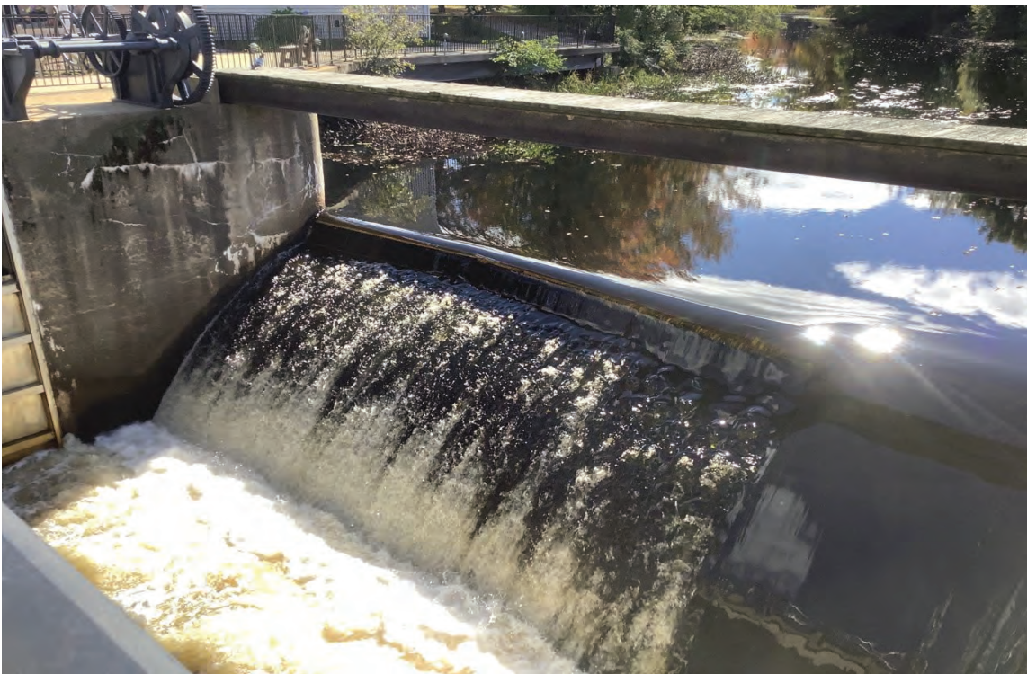
Photo 8: View south of the Contoocook River Dam spillway. 10/07/2021.
